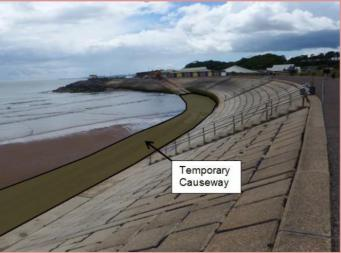
The recovered stone is initially being used to form a temporary causeway between the slipway and groyne 1. This will allow a longer tidal working window and help the work to be completed in a timely manner. The steel mesh baskets and stone are being separated at source to allow the separate materials to be reused and recycled.
